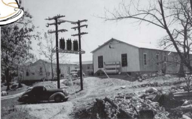
PEC's First Substation at Walter Graper's Fittstown, Oklahoma (1938)
